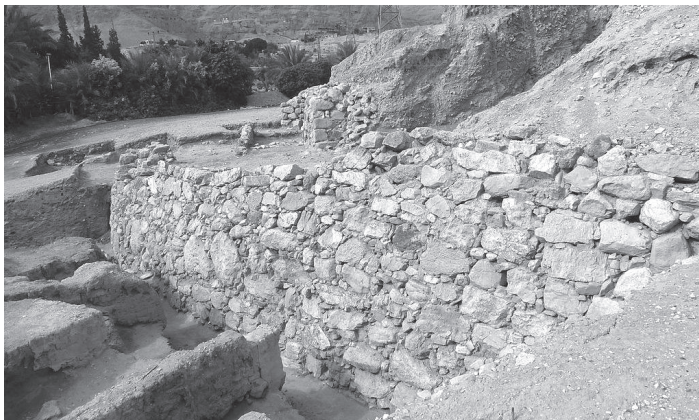
Segment of the stone retaining wall located at the archeological site of Jericho.
